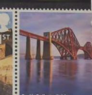
Forth Railway Bridge
